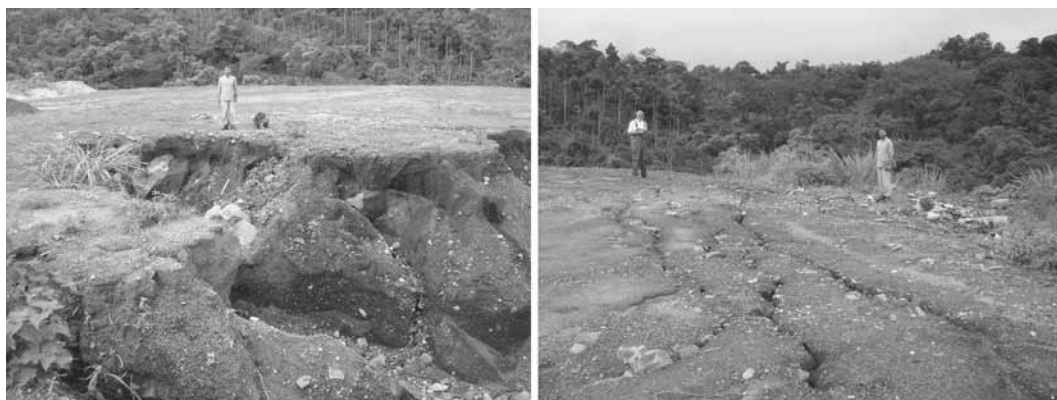
Fig. 3: Landfills and dumps in the area where collapse and cracks were observed.
