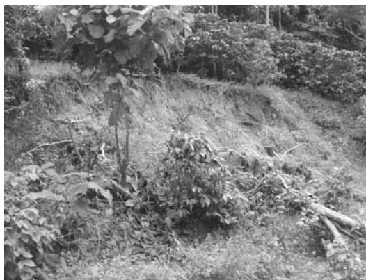
Fig. 2: Small mass movements in the artificial road cuts of the area.
