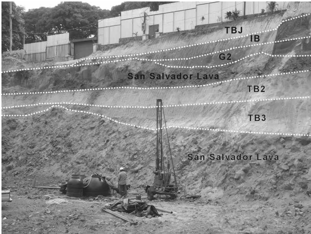
Fig. 10. Almost complete stratigraphy of the San Salvador formation; photo for reference was taken about 3 kms north of the studied area during the beginning of engineering geology mapping.
